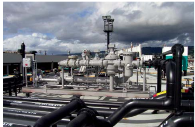
Barge mounted in-line blender with viscosity control
